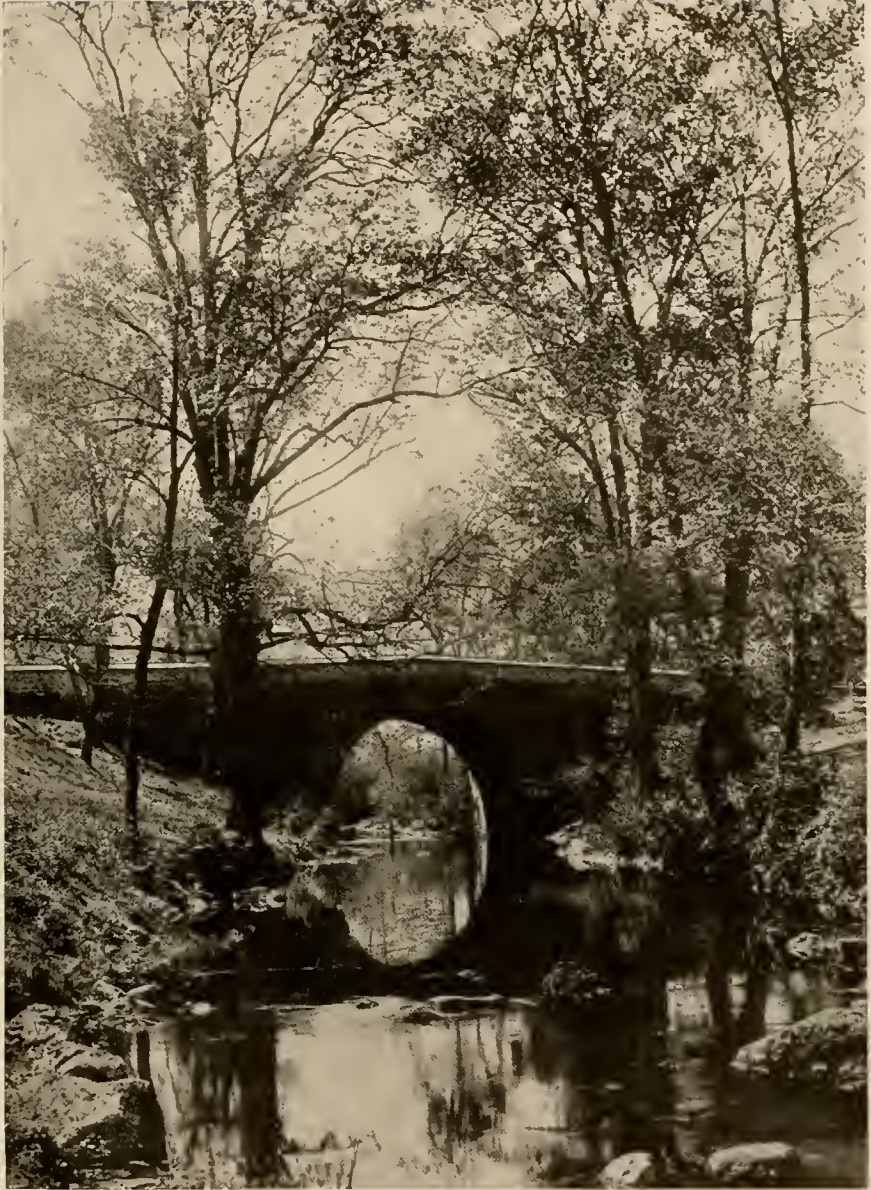
OLD BRIDGE OVER CRESHEIM CREEK.
